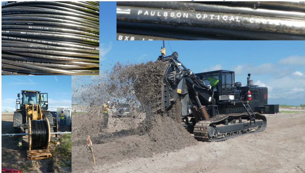
Installation of a 2.7 km optical DSS, DTS & DAS Cable to a depth of 14 ft
