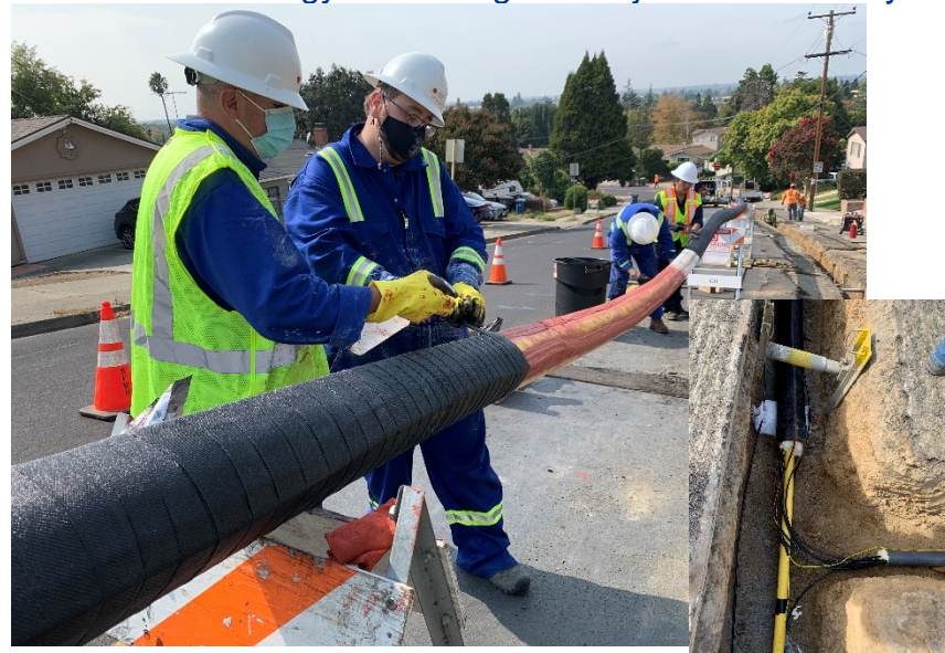
Installation of Optical Cables on a Pipeline @ Hayward Fault
