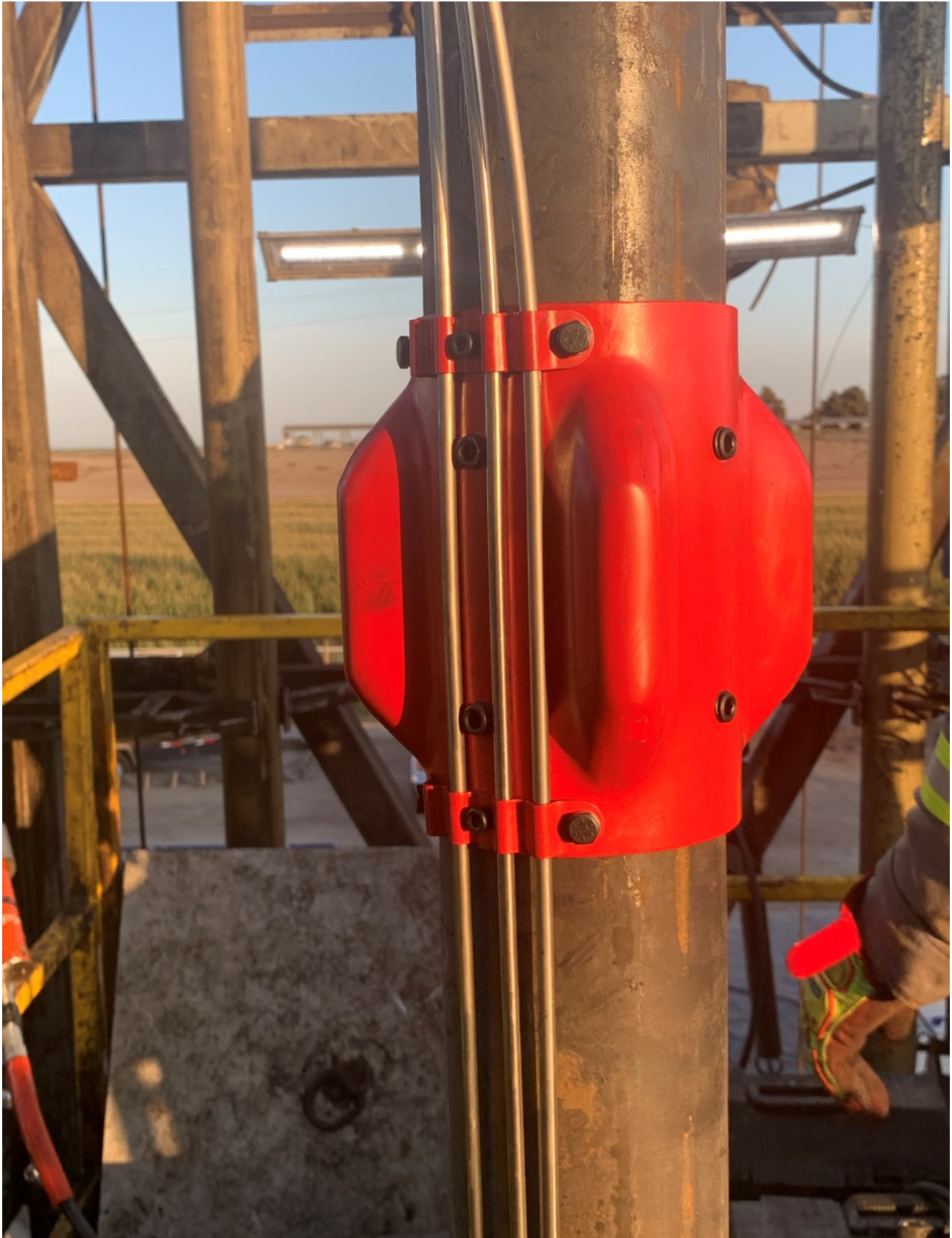
Figure 6. This figure shows the 4.5" OD production tubular that serves as a carrier of the optical fiber encapsulated in the 1/4" stainless steel tubing. The 1/4" tubing is secured to the 4.5" production tubular using a specialized centralizer that secures and protects the 1/4" tubes containing the fiber.
